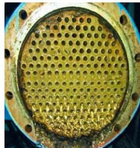
Scaling in a shell and tube heat exchanger due to poor water treatment practices.
