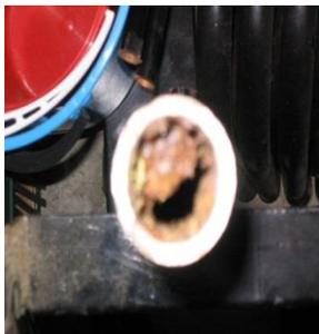
Corrosion inside package unit due to poor water treatment practices
